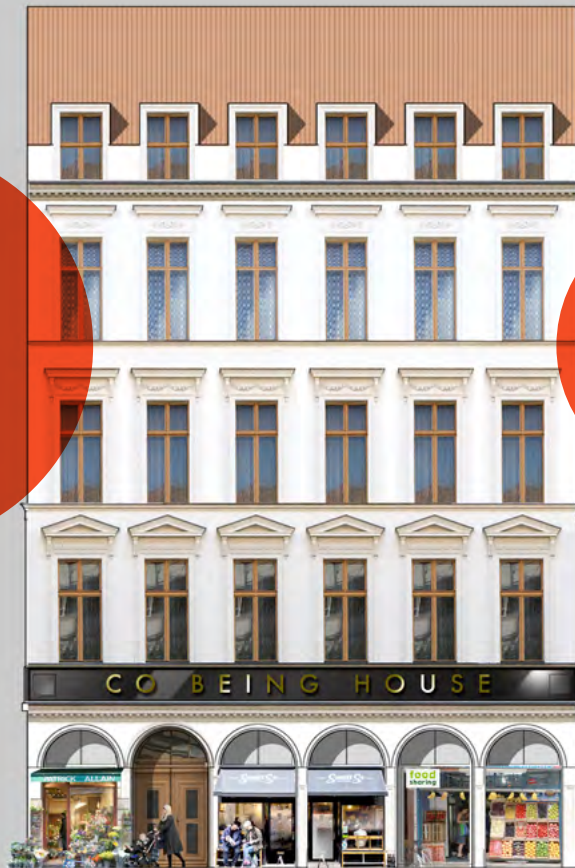
Co-Being House Facade (Vienna Style)
